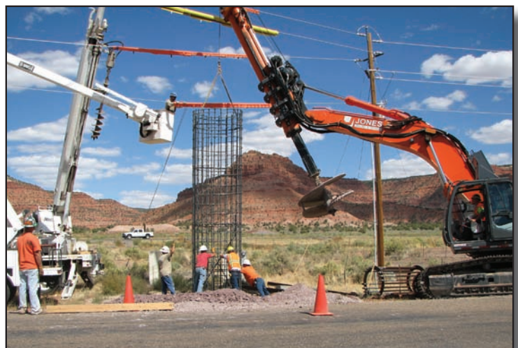
- Kanab 400 South Transmission Line Work -
