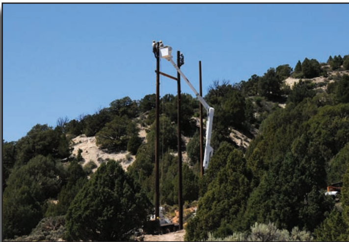
- Hatch to Tod's Transmission Line Work -
