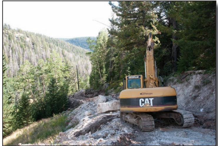
- Barney Top Underground Line Work -
