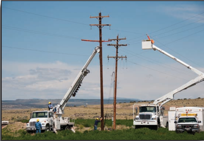
- Line Work Near Bicknell -
