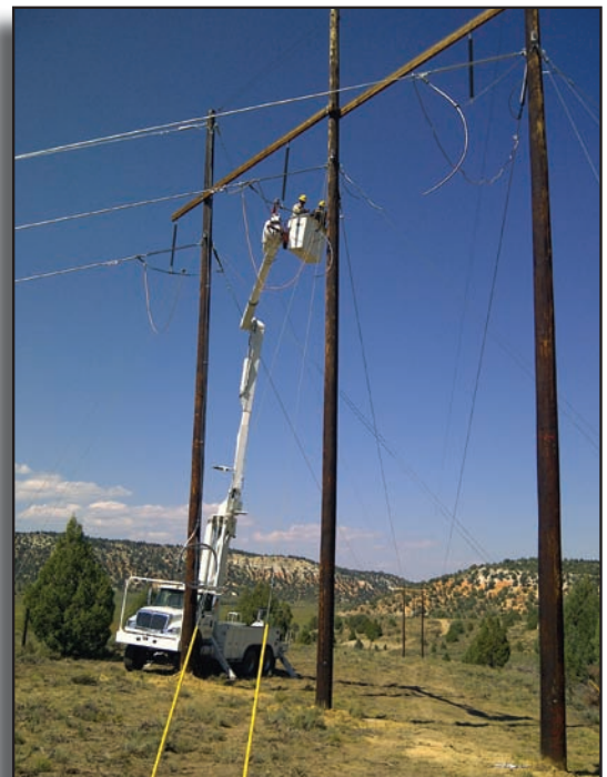
- Hatch to Tod's Transmission Line Work -
