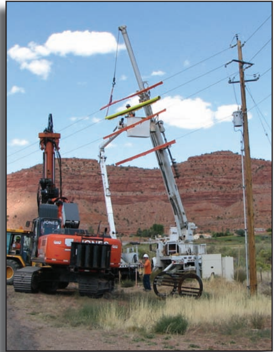
- Kanab 400 South Transmission Line Work -
