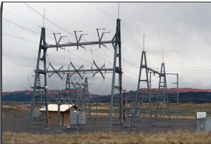
- New Hatch Substation -
