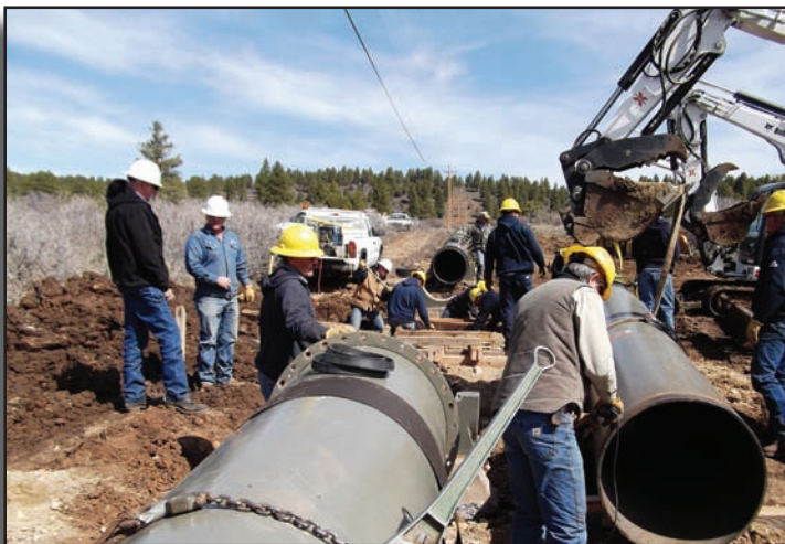
- Repairs to Penstock Near Boulder Plant -
