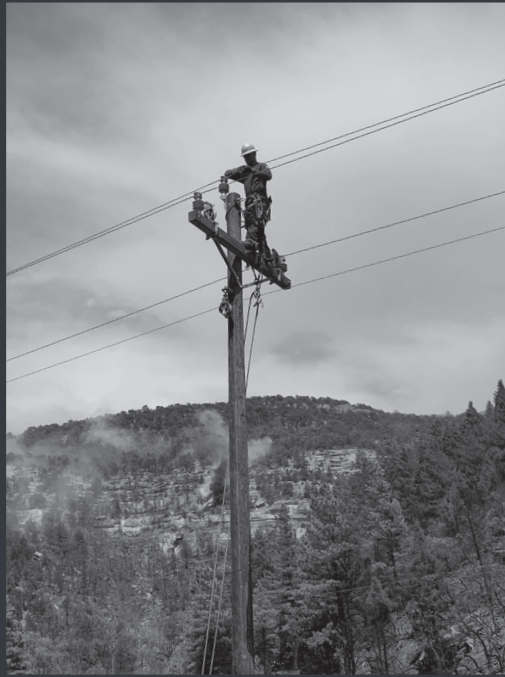
CREWS ON THE KAIBAB MTN.
