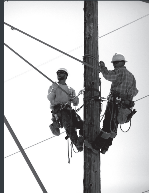
REPAIRING A LINE
