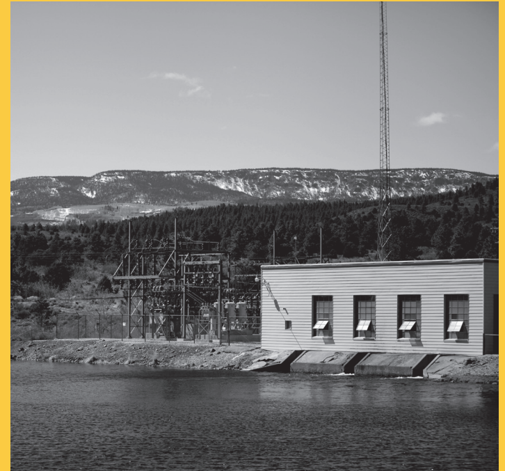
BOULDER HYDRO FACILITY
