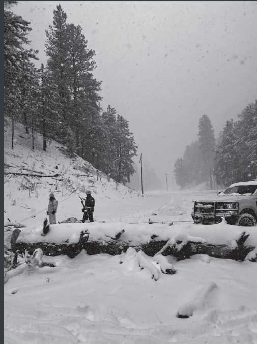
REMOVING A DOWNED TREE ON A LINE
